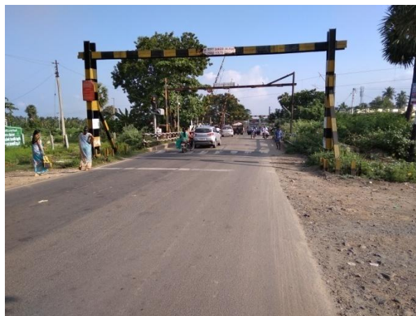
Railway level crossing at km 0/250 of SH 222
