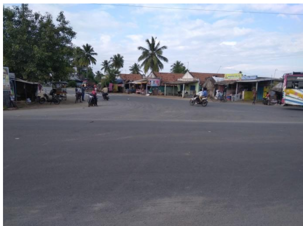
Built up at start point at km 0/000 of SH 222
